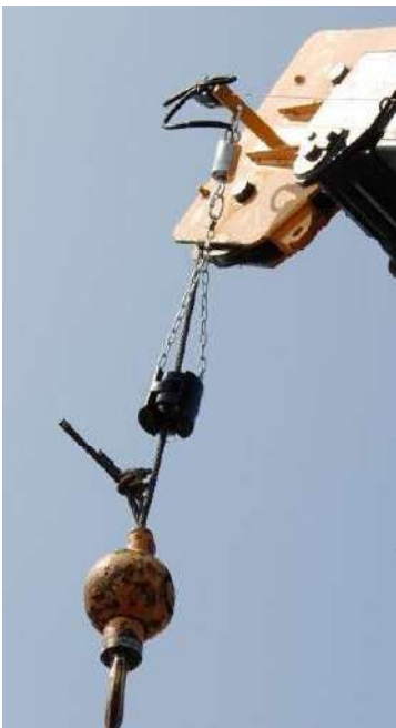
ATB switch with weight and chain assembly
